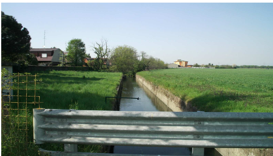
Fig. 6 – Torrente Guisa in Via Vismara vista nord.
